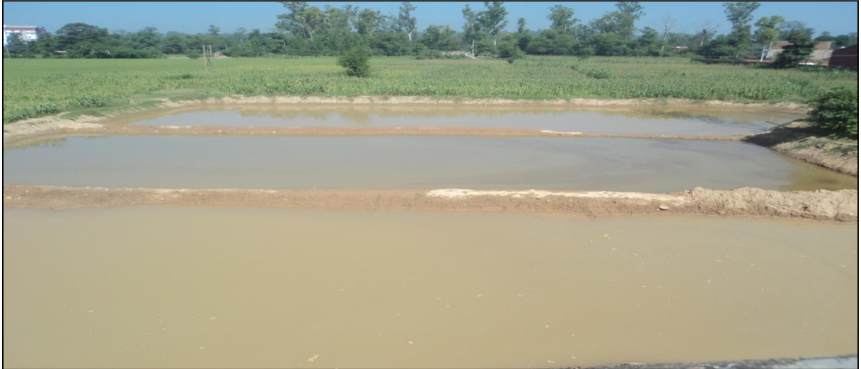
Fig. A view of nursery ponds constructed at Fisheries estate Ratyod.
